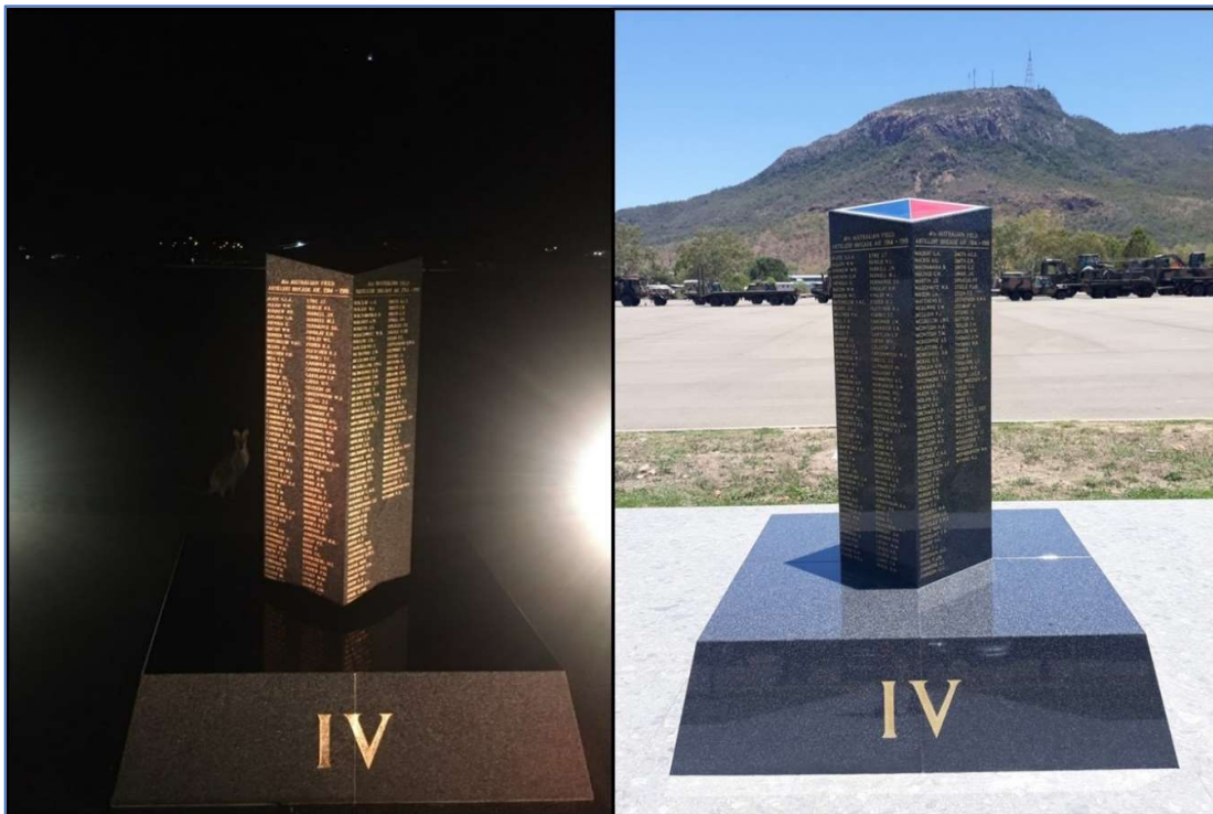
The completed Memorial Night and Day view prior to any landscaping work
